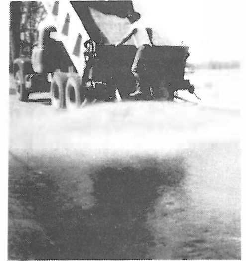
TAVERN ROAD JUST HAD SEAL-COATING BY COUNTY ROADMEN WHO KEEP ALPINE'S STREETS IN FINE CONDITION. ABOVE BIG TANKER SQUIRTS WARM OIL ON ON HALF OF STREET.
